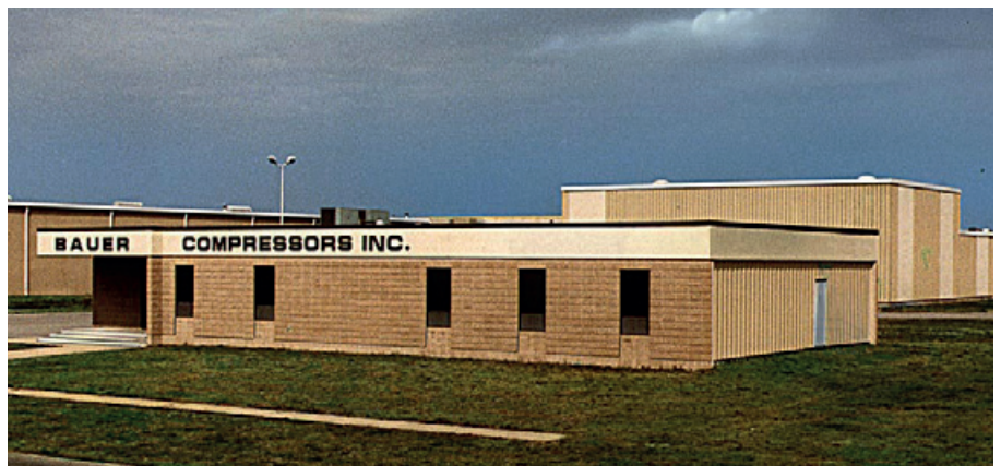
The new BAUER plant in Azalea Garden Road, Norfolk, Virginia
