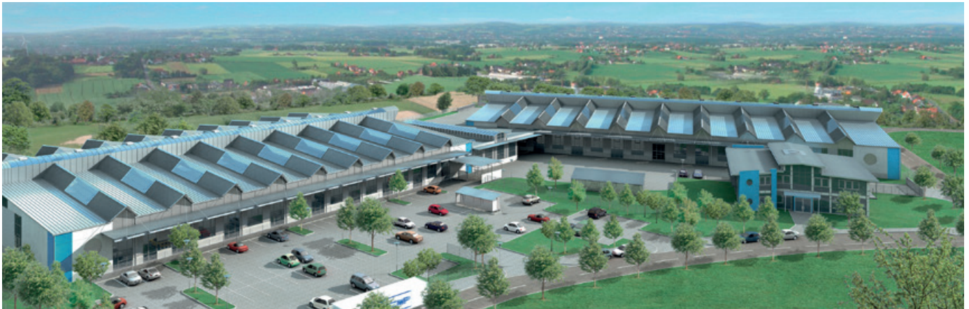
A second production hall enabled capacity to double.
